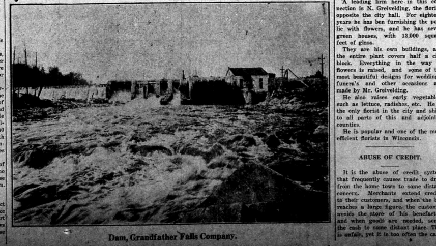
Dam, Grandfather Falls Company.
