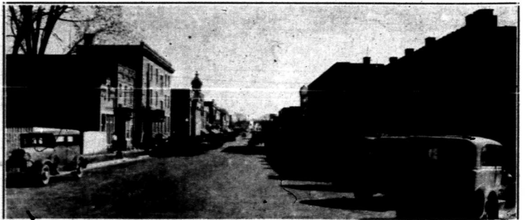
Looking east from Arverson's garage on the corner of Scott and East Main. The courthouse, whose tower shows above the Citizen's American bank building in left center, is three blocks down, while the street for two blocks further is devoted entirely to business buildings.
