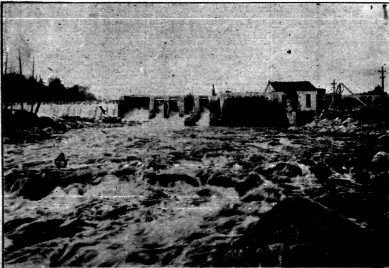
Grandfather Falls Dam, situated about 14 miles northwest of Merrill is one of the several large water power developments in the county. This dam furnishes power to one of Merrill's leading institutions, the Grandfather Falls Co.
