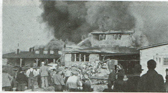
Merrill Box Company destroyed October, 1938.
