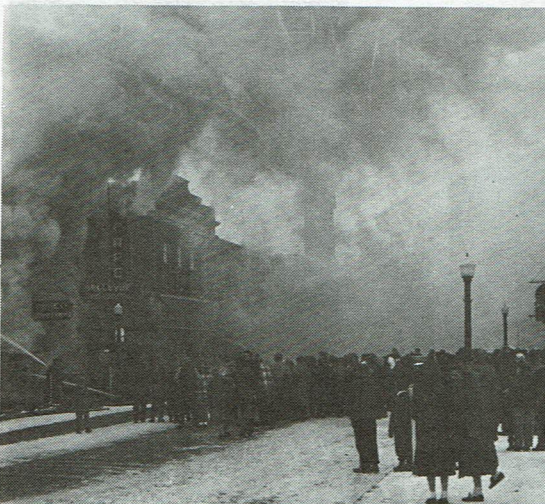
Mead's Store, (site of new "The Guy's" store) gutted in November, 1951.
