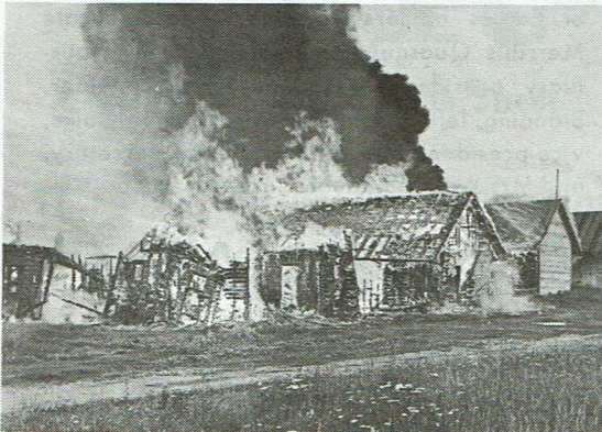
Lincoln Co. Fairgrounds mostly destroyed July, 1943.
